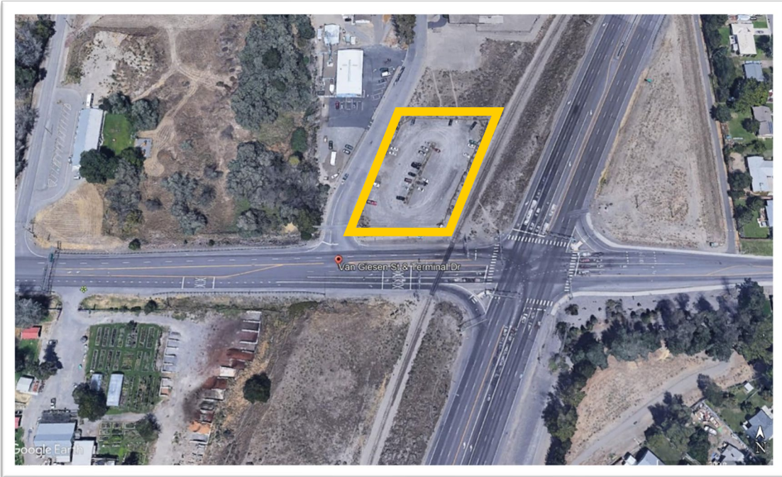
Figure 17: Terminal Drive Park & Ride (SR 240 & SR 224 Van giesen)
